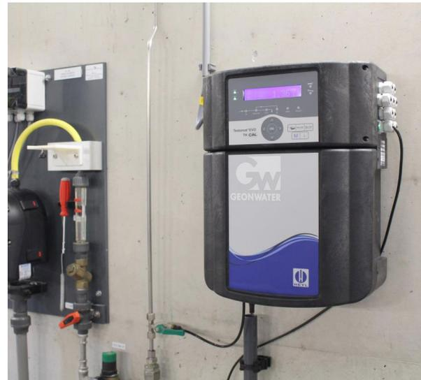
Our customers of Geonwater B.V./Netherlands use the Testomat® EVO TH CAL to measure water hardness. They particularly appreciate the calibration function of the device.
